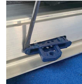
4. Pry the housing out using a screwdriver
