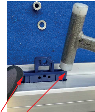
5. Insert the new Klick-Klack locking mechanism in the correct position in the slotted hole and alternately hammer left/right with a rubber mallet
