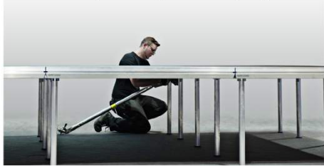
Attachment of Layher alu diagonal brace, bay height 0,475 m
