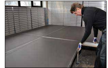
hook tongue profile into groove profile
