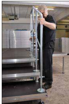
assemble stairway rail, mount it on bolts and fasten safety screws
