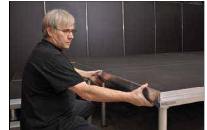
direct attachment of lining lath
