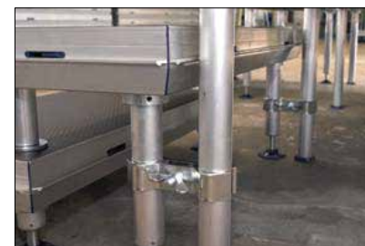
connection tongue profile: 2 leg links 110 mm
