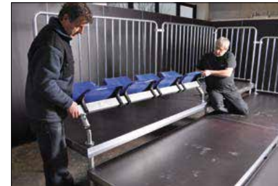
put on seat girder and secure it
